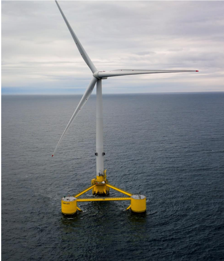
Credit: Photo of the Kincardine Offshore Wind Farm project courtesy of Principle Power
